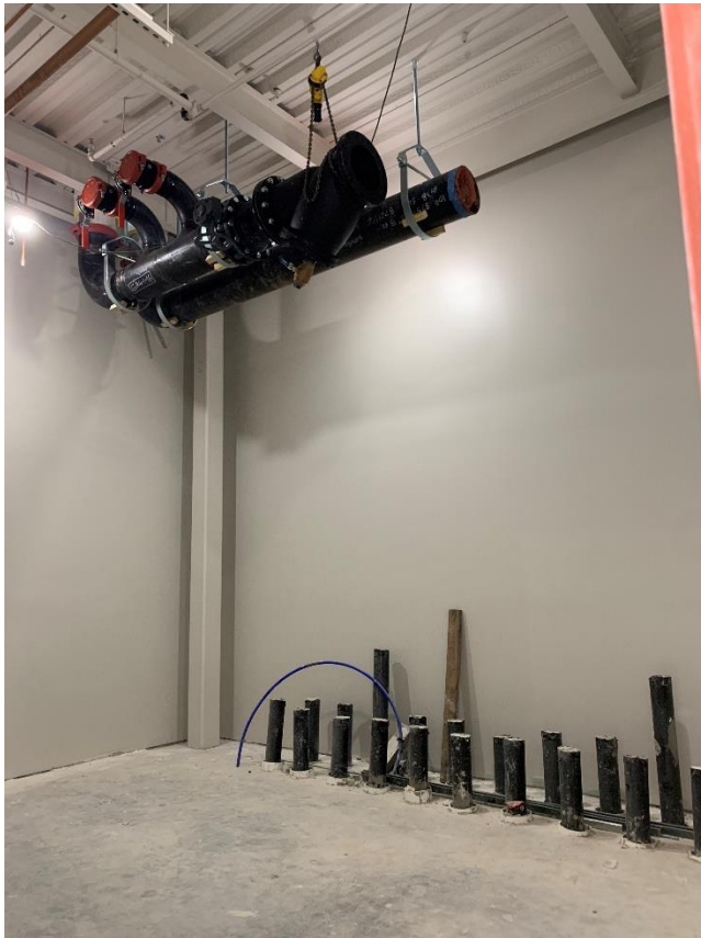
16. Area 6 First Floor – Manifold room geothermal equipment installation in progress.
