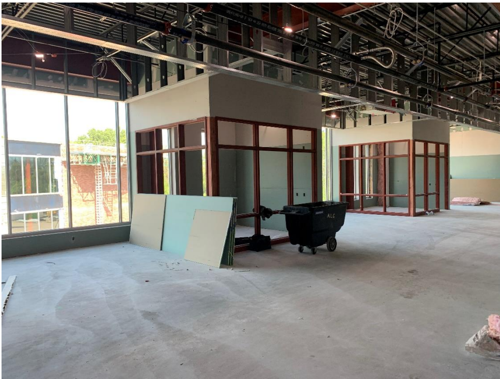
20. Area 5 Second Floor – Interior gyp board installation in progress.
