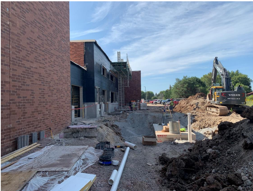
10. Area 3 West – Below grade work in progress. Exterior brick veneer and cast stone panels installed.
