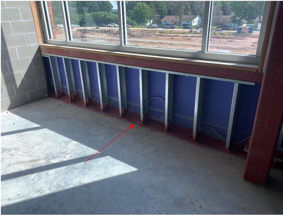
21. Area 6 Second Floor - Fire safing insulation.
