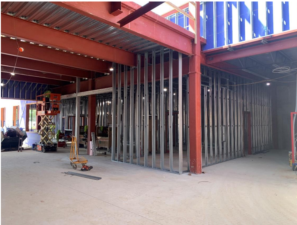
32. Area 1A/2B First Floor – Interior metal stud framing installation progress.
