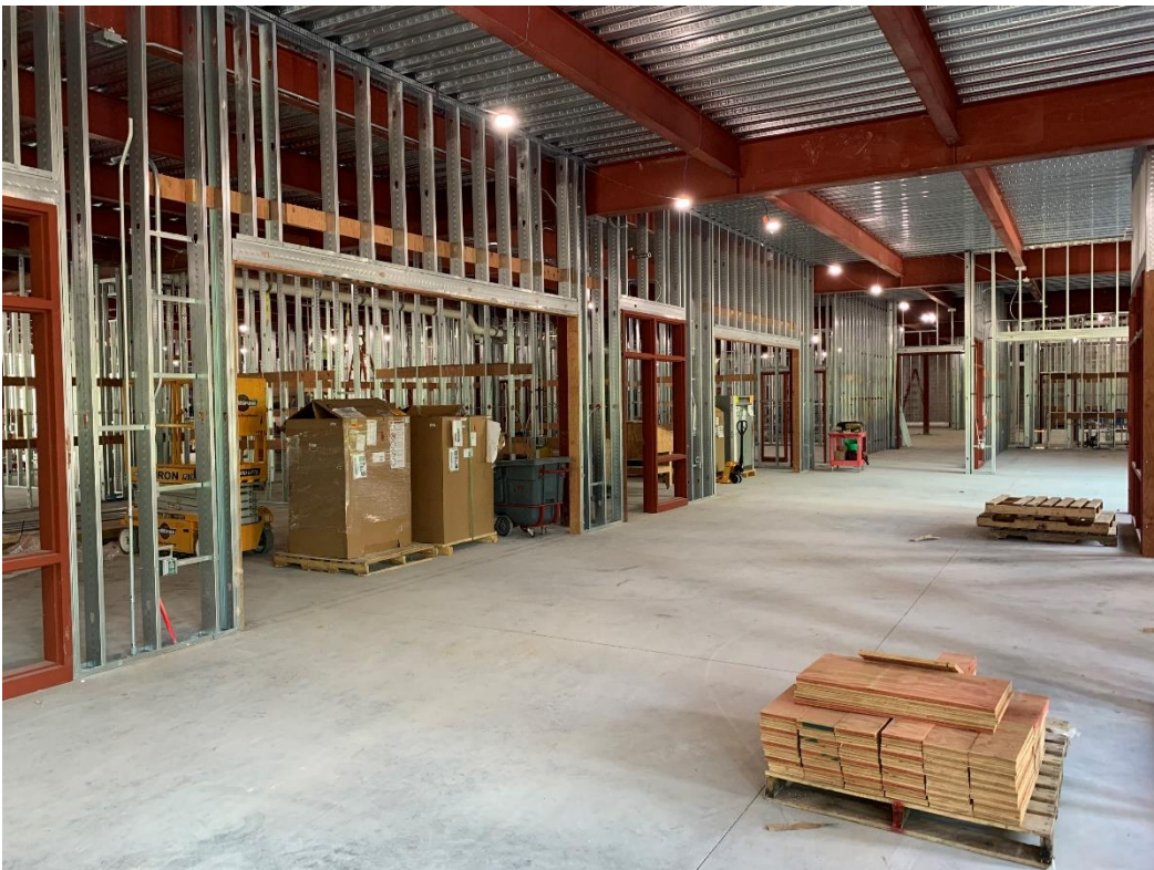
24. Area 4 First Floor – Metal stud framing and blocking installation in progress.
