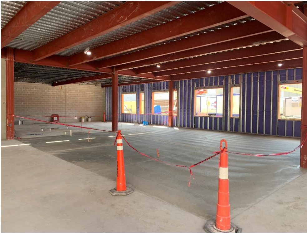
32. Area 1A/2B First Floor – Interior metal stud framing installation progress.
