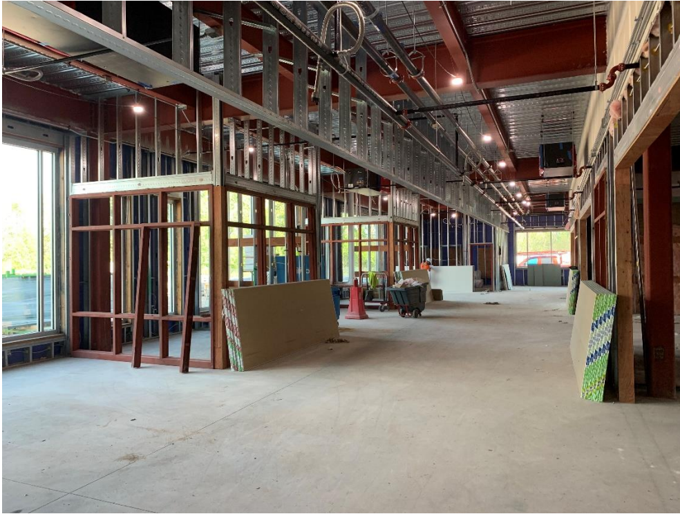
20. Area 5 Second Floor – Interior gyp board installation in progress.
