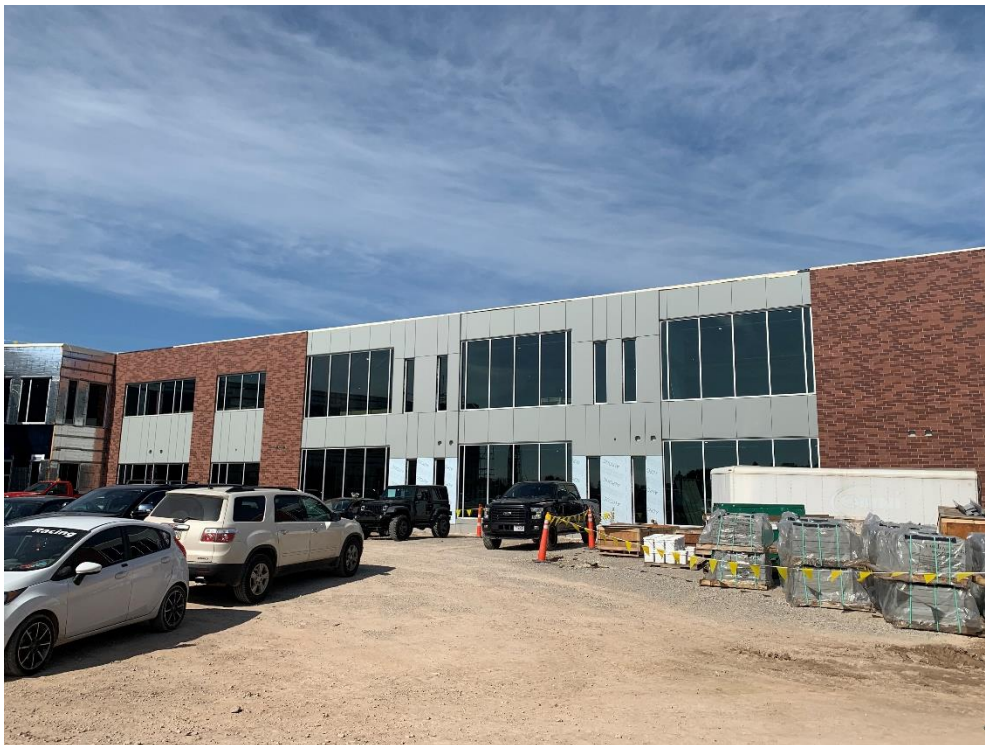
4. Area 5 East – Composite metal panels installed.
