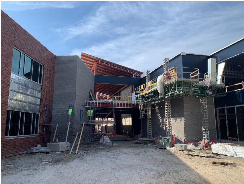
6. Area 1B North – Exterior brick veneer installation in progress.
