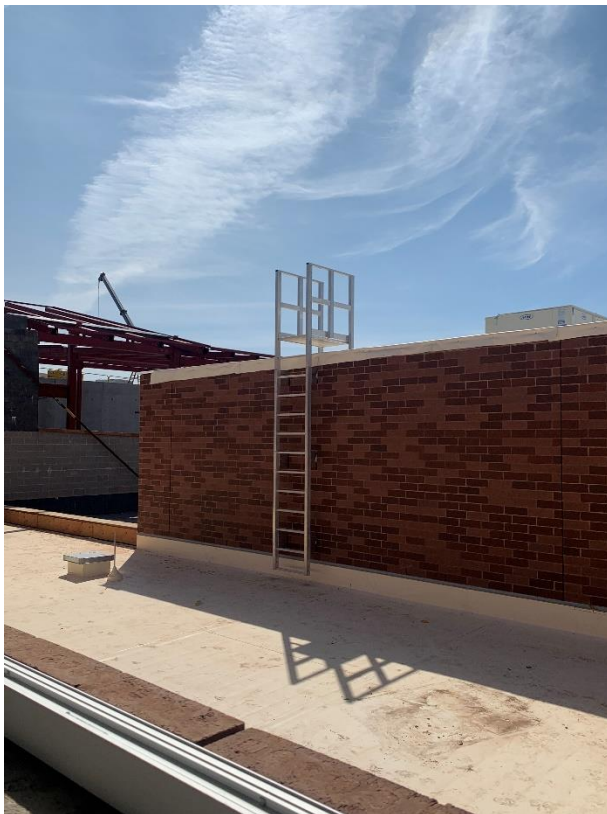
30. Area 2 - Roof Ladder and roofing installed.
