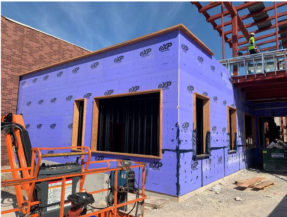
12. Area 1A South – Exterior sheathing, window blocking, and weather proofing membrane installation in progress.
