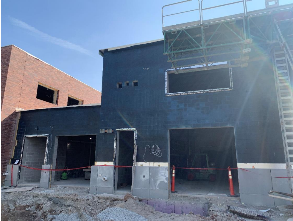
12. Area 1A South – Exterior sheathing, window blocking, and weather proofing membrane installation in progress.
