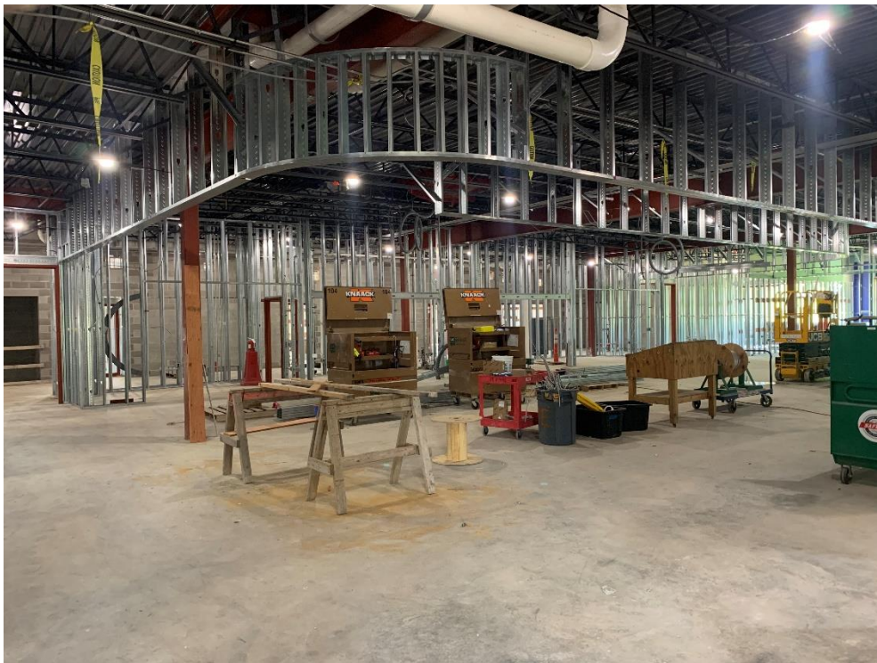
28. Area 3 Second Floor – Interior metal stud and soffit framing in flex café in progress.
